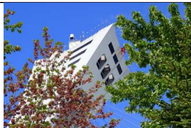
Olympic stadium tower and botanical garden
